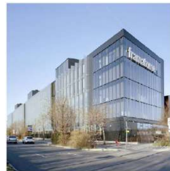
WORK IN PARK Lyon, France
