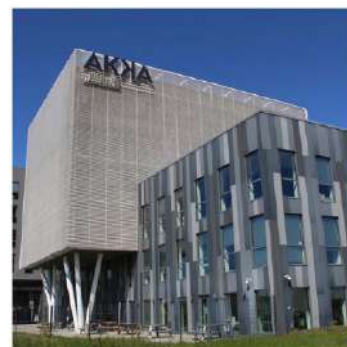
AKKA Montigny-le-Bretonneux, France
